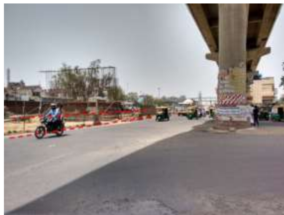
No permanent barricading – concrete barricades are placed sparsely
