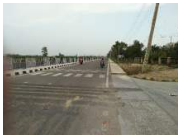
Exhibit 36: Rumble strips on NH as a Traffic Calming Measure but not as per IRC standards
