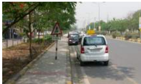
Exhibit 22: Warning Sign installed but not maintained which has resulted in wrong orientation of sign.
