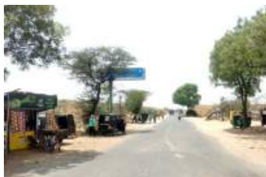
Exhibit 6: Visibility of overhead information sign board obstructed by tree on highway
