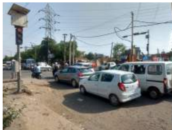
Exhibit 10: Height and location of a primary Traffic Signal on intersection not in compliance with IRC standards
