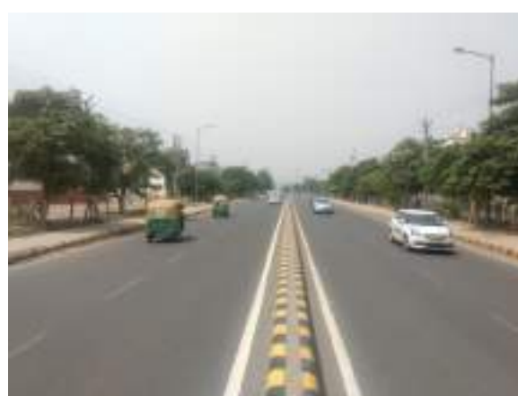
Exhibit 8: Pavement Markings present and adhering to IRC Code on urban roads
